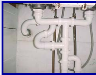
AMATEUR PLUMBING INSTALLED?
