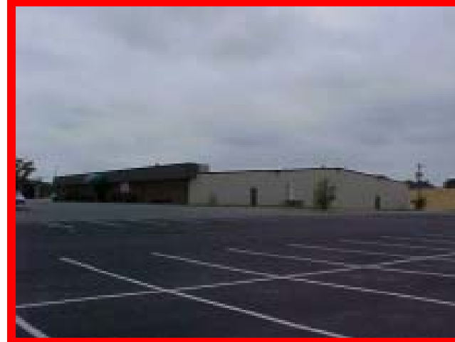
23,000 S.F. 631 Cinema Dr., Kernersville, NC PIEDMONT LANES BOWLING ALLEY
